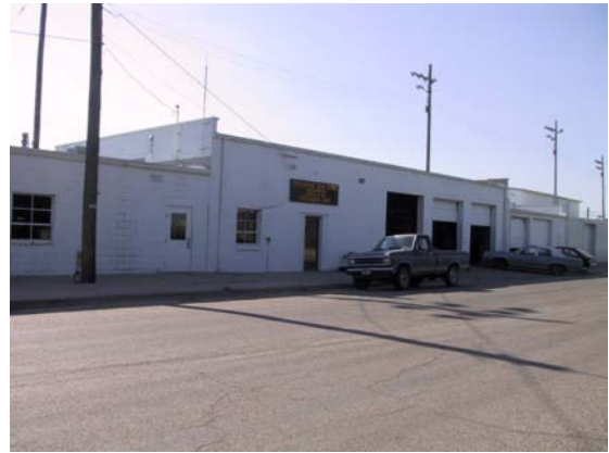
Torrington High School Auto Mechanic Shop
